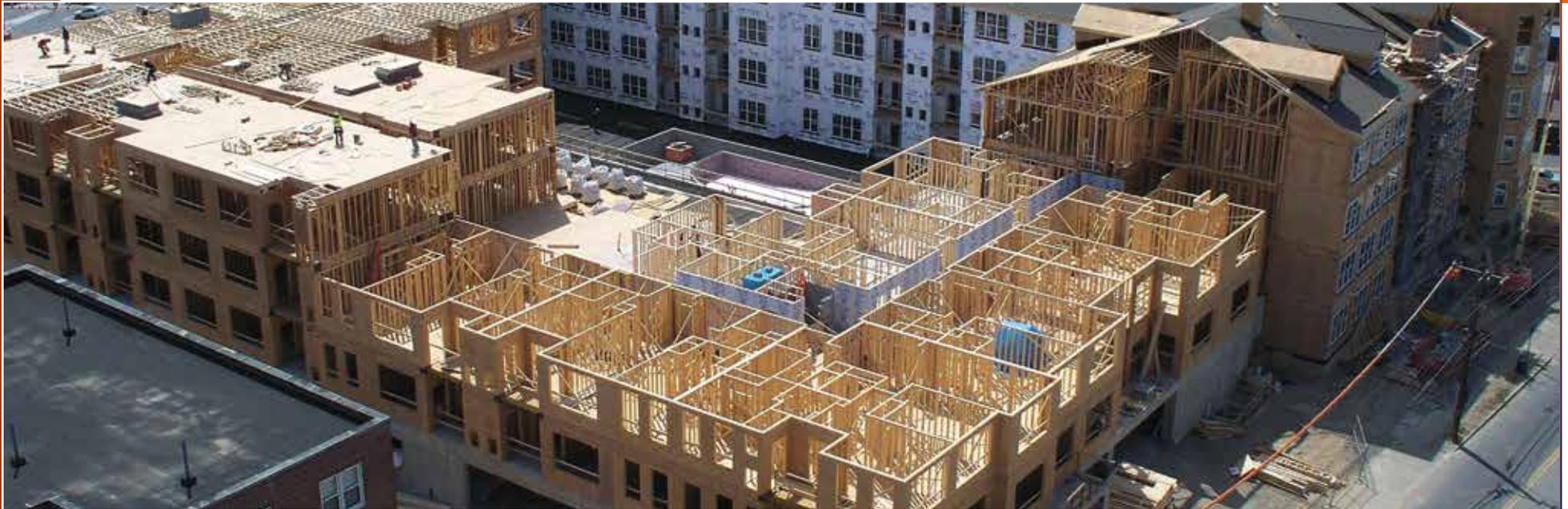
*Multi-dwelling construction with a lightweight prefabricated frame
